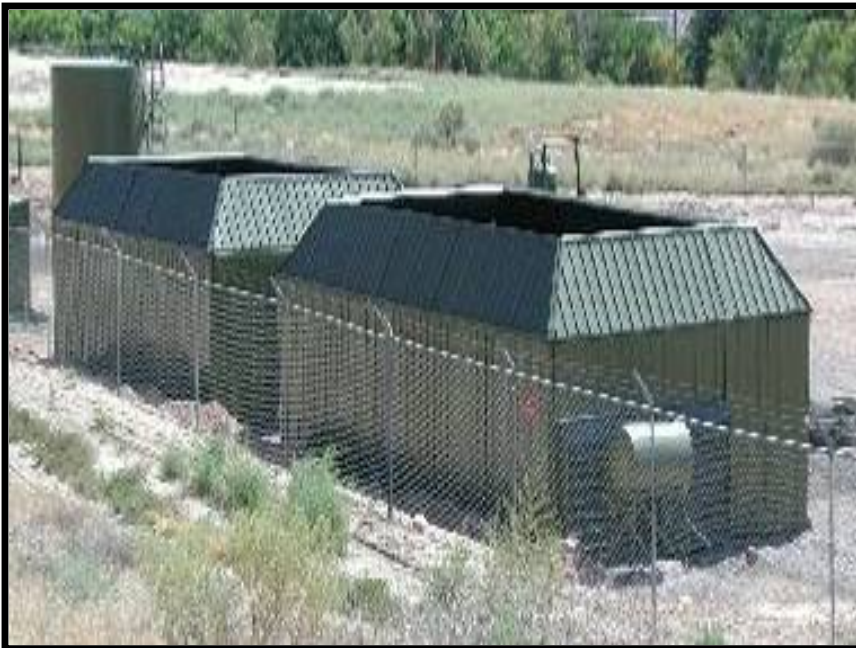
4-Side, Open Compressor Building
