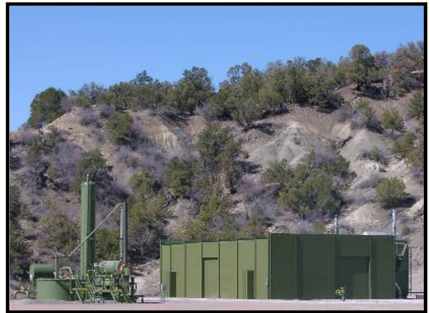
4-Side, Closed Compressor Building
